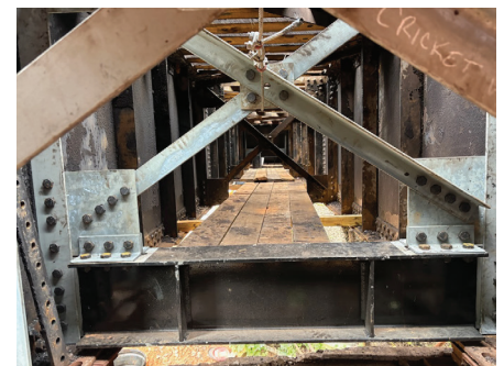
Jacking Beam Install
