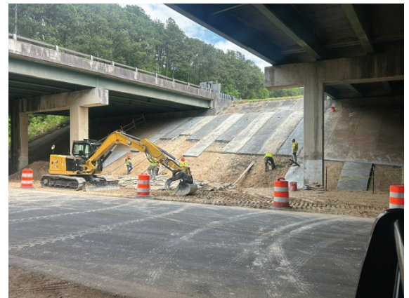
Job #26015 - Slope Paving Repair
