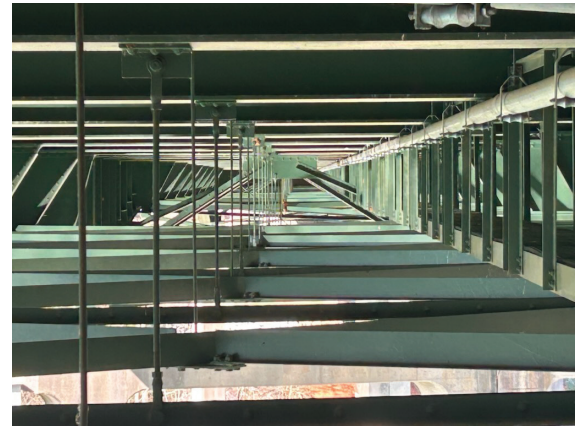
Job # 25055 – Steel Repairs
