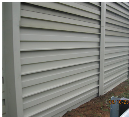
Job #26038 - Sound Wall (After)
