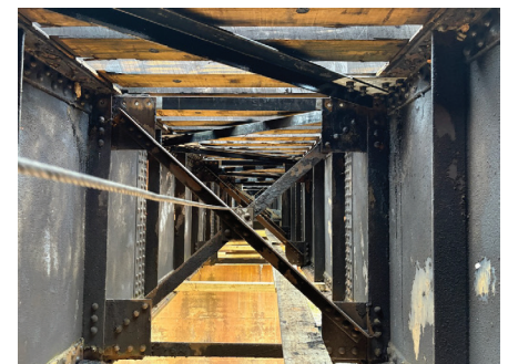
Misc. Steel Repairs
