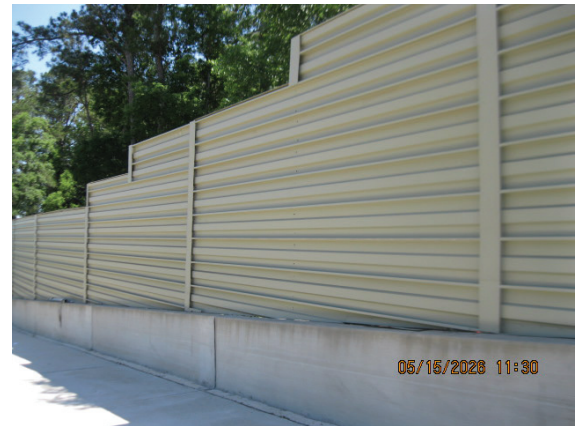
Job #26014 - Sound Wall (After)
