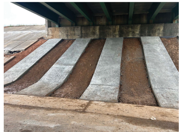
Job #26025 - Slope Paving Repair
