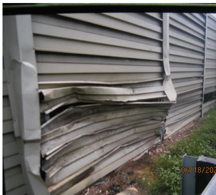
Job #26038 Sound Wall (Before)
