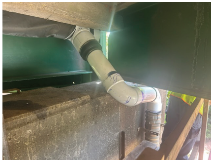
Job #25055 – Drainage Repair
