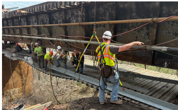
Flange Angle Replacement, Spartanburg SC
