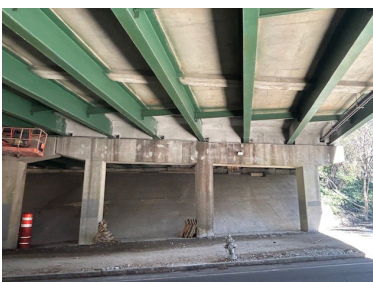
Project #25078 - Completed Edge Beam
