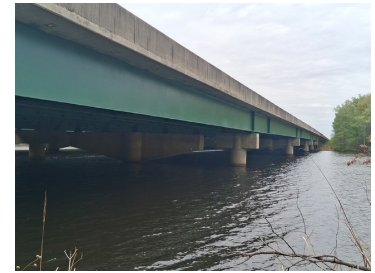
Project #23129 - Bridge Paint
