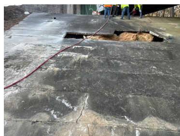
Project #26015- Slope Paving Repair
