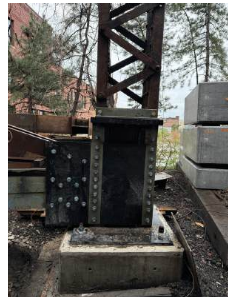
Completed Column & Precast Pedestal Replacement
