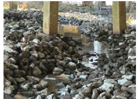
Project #23129 - Rip Rap
