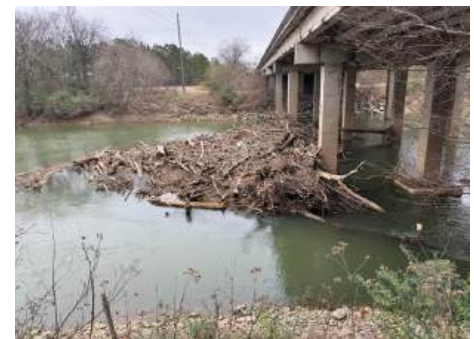
Project #25001 - Rome Debris Removal
