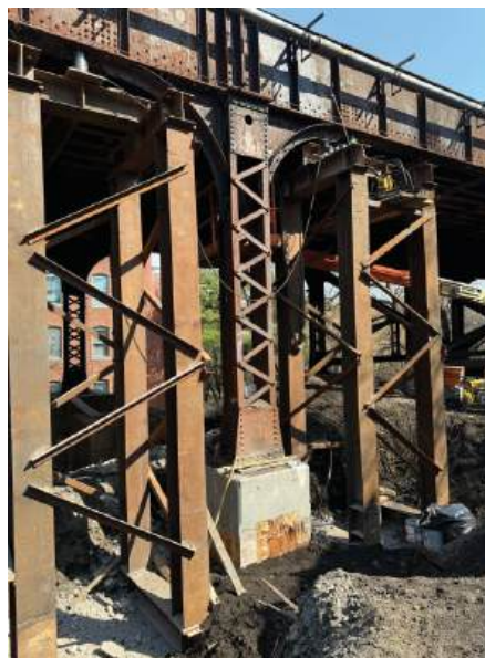
Jacking System for Column & Precast Pedestal Replacement
