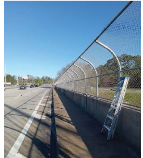
Project #23107 - Fence Repair
