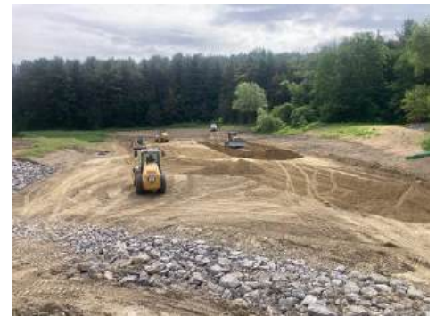
Final Grading Around Spillway
