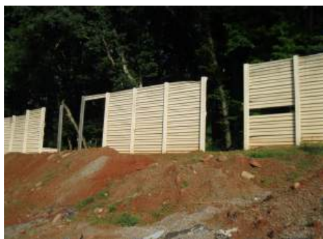
Project #25036 – Sound Wall
