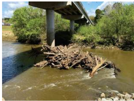
Project #25031 – Canton Debris Removal
