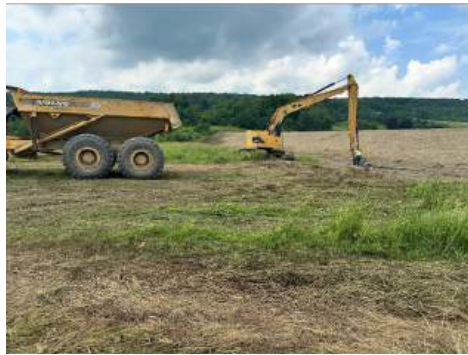
Top Soil Stripping
