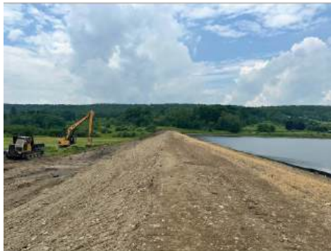
Placing Embankment Material Buildup
