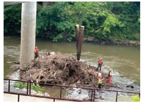
Project #25031 – Canton Debris Removal
