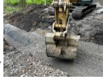
Culvert Replacement in Lockport, NY
