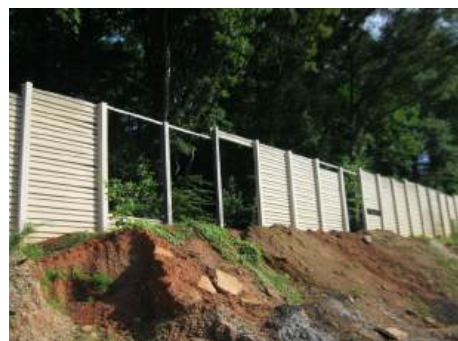
Project #25036 – Sound Wall
