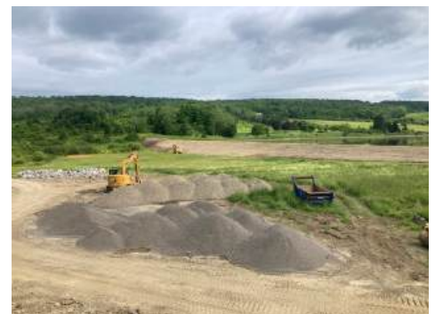
Access Road and Dam Rehabilitation
