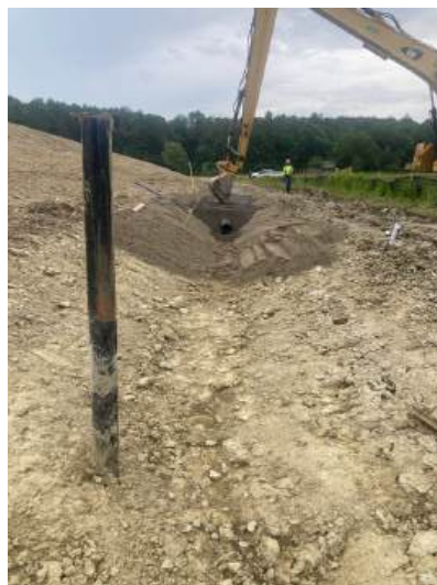
Installing Drains at Toe of Levee
