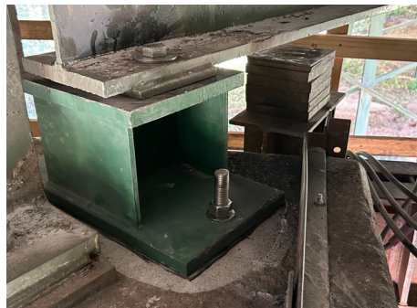
Project #24076 – New Bearing
