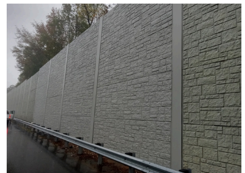
Project #24074 – Wall Repair Complete
