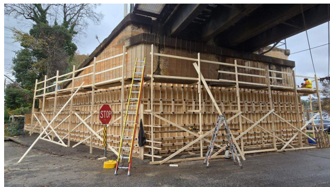
Spartanburg, SC - Abutment Encasement
