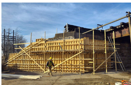
Bridge Replacement - Millersburg, IN
