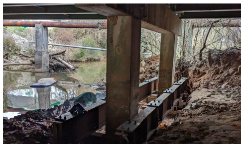
Bent 2 - Constructing Falsework
