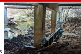
Project #23002 – Falsework Begun
