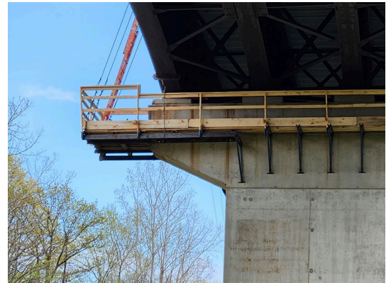
Scaffolding System Used To Access The Piers
