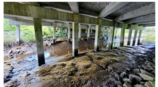
Project #23070 – Liberty County Piles To Be Encased
