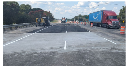
Project #23073 – Approach Slab
