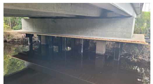
Project #23080 – Pier Cap Reinforcement
