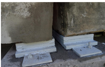
Project #23080 – Jacking Finished Product
