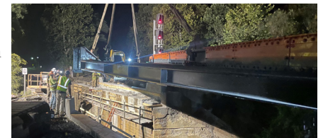
Span Replacement in Burkeville, VA
