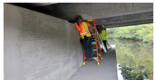
Project #23080 – Joe Howland With The Jacking Crew
