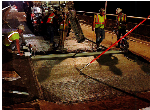
Crew Working Late At Night Utilizing The Roller Screed.
