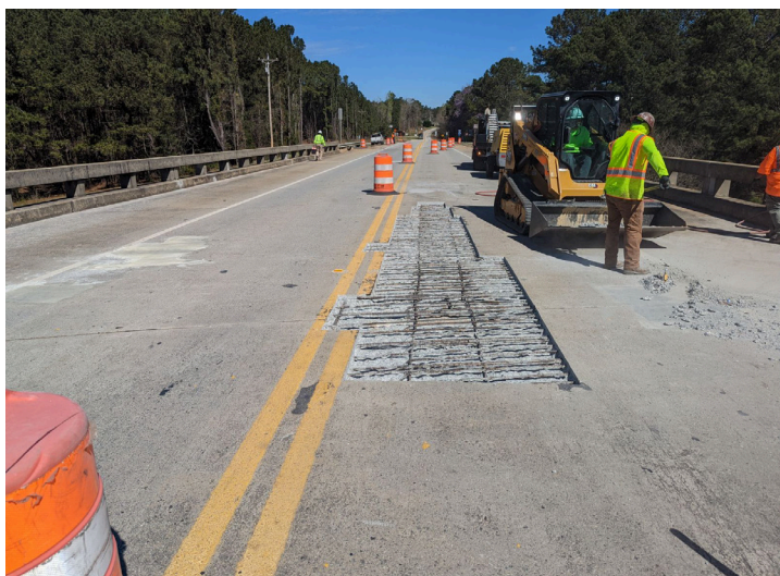
Concrete Deck Patching
