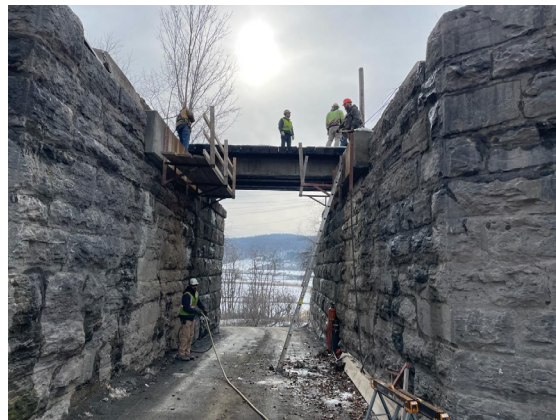
Span Replacement in Richmondville, NY
