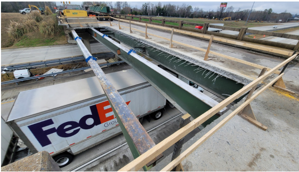
Overhang and Deck Removal Complete
