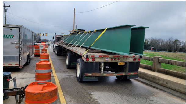
New Steel Beam
